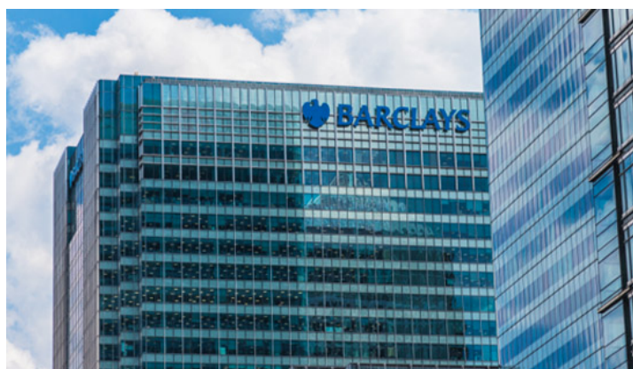
Barclays Bank Building
