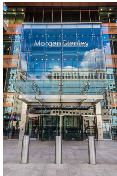
Morgan Stanley Building
