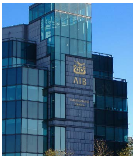
Allied Irish Banks Building
