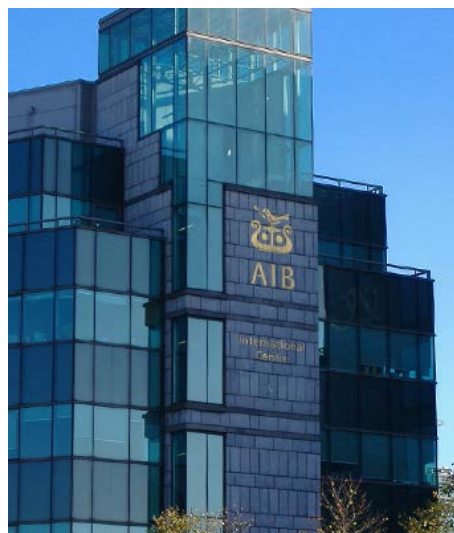
Allied Irish Banks Building
